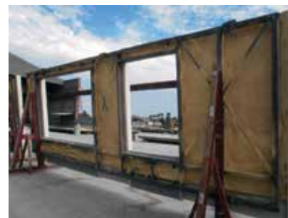
Interior Panel View with Spray Foam Insulation ©Clark Pacific 2013
